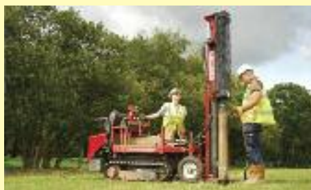
Sinking one of the series of boreholes. Photo by Gareth Owen / CCW
